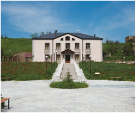
New Community Center in Talish
